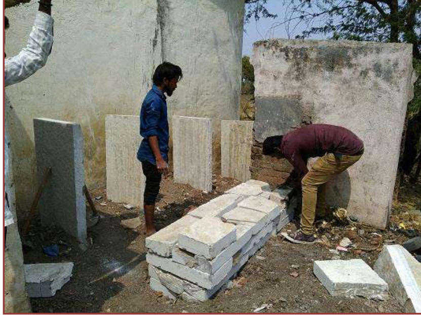
Students constructing toilets for students in Govt. School, Tonasanahalli(s)
